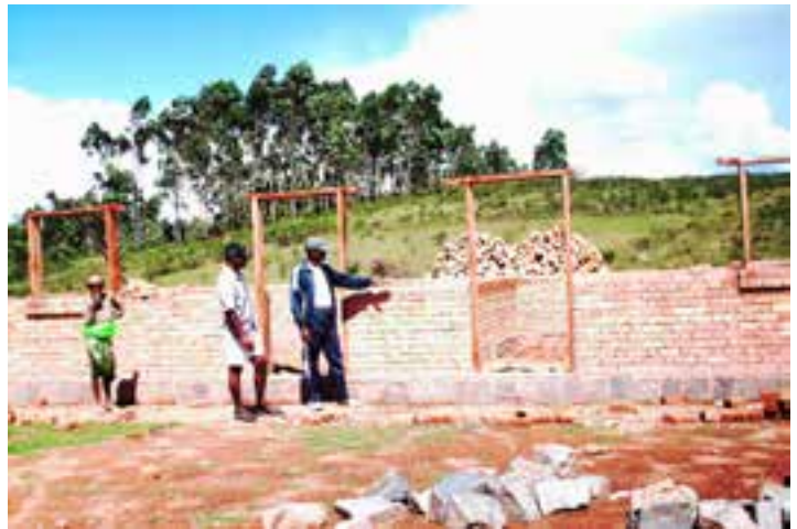
Fig. 3. School construction under progress.
